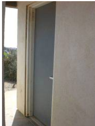
Location: Men's Restroom Photo # 50
