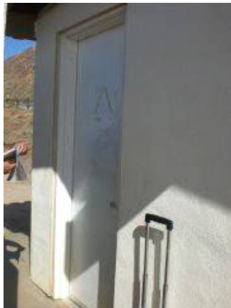
Location: Women's Restroom Photo # 34
