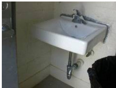
Location: Men's Restroom Photo # 51
