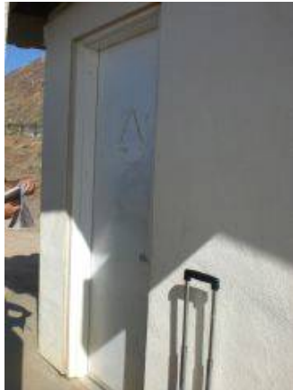
Location: Women's Restroom Photo # 34
