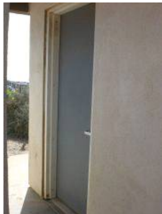
Location: Men's Restroom Photo # 50
