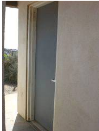
Location: Men's Restroom Photo # 50
