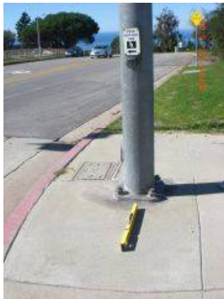
Location: Crest Rd. & Hawthorne Blvd. Photo # 107
