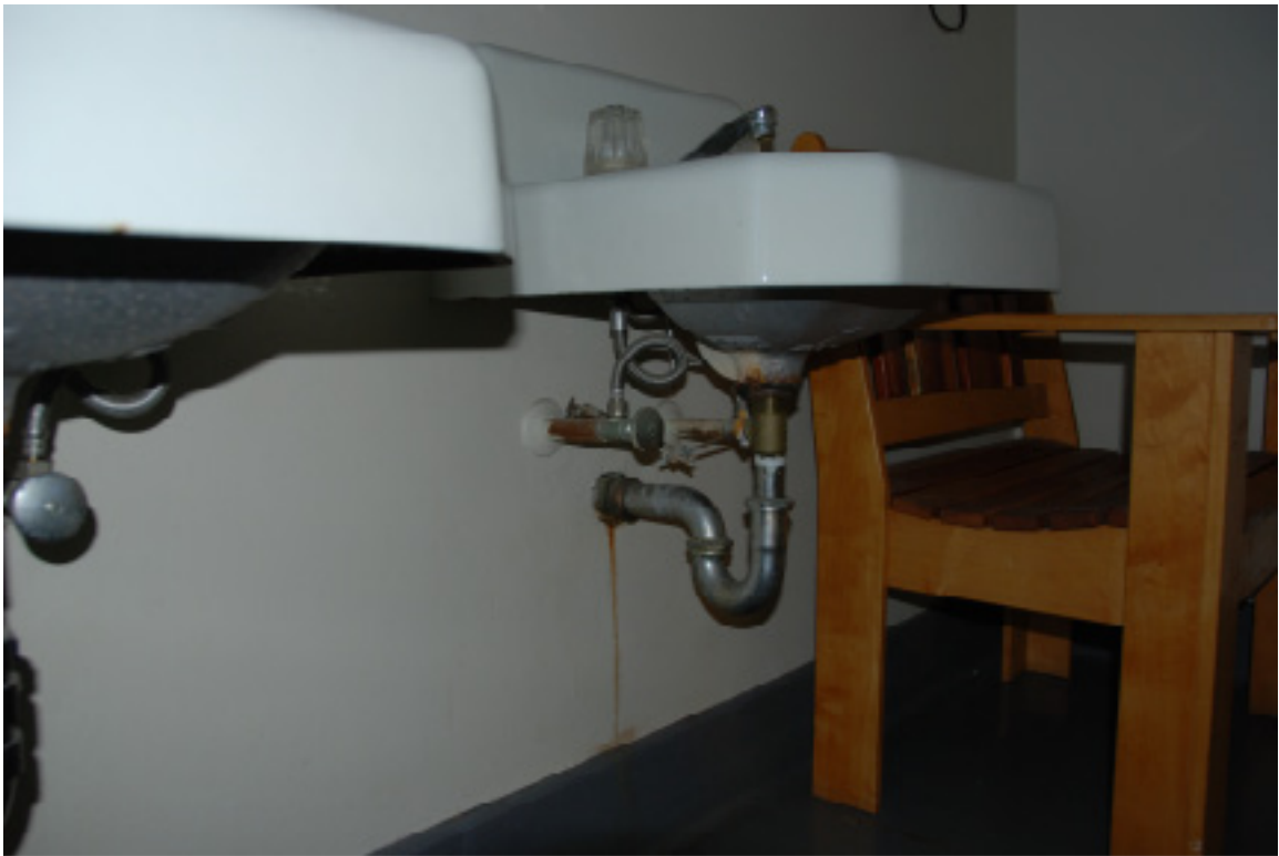
Leaking Plumbing
