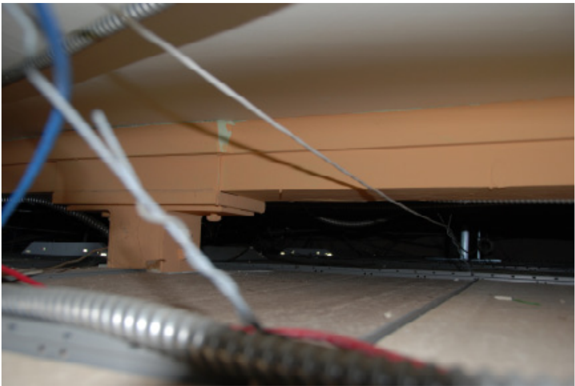
Space Above Ceiling
