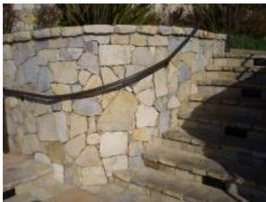
Location: Stairs Photo # 35
