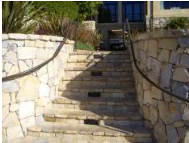
Location: Stairs Photo # 33
