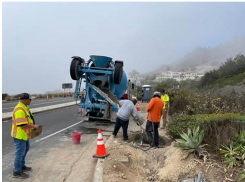
Concrete was poured for most of the pole foundations last Friday, and work continues this week digging the remaining foundations for the new traffic signal project at the intersection of Palos Verdes Drive South and Palos Verdes Drive East. The remaining concrete foundations are expected to be poured this Friday.
