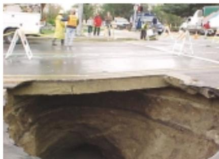
drain pipe. The pipe was located far below the street, so when it failed, the roadway collapsed as well. The resulting sinkhole was large enough to swallow a dump truck. The adjoining sewer system, serving thousands of homes in the area, was also at risk of collapsing.
