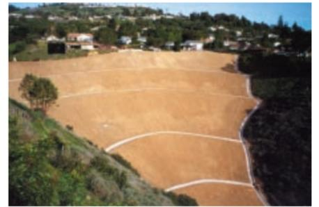
reconstruction and vegetation restoration. The project repaired the erosion-damaged canyon slope, aged storm drain system and remediated an active landslide.
