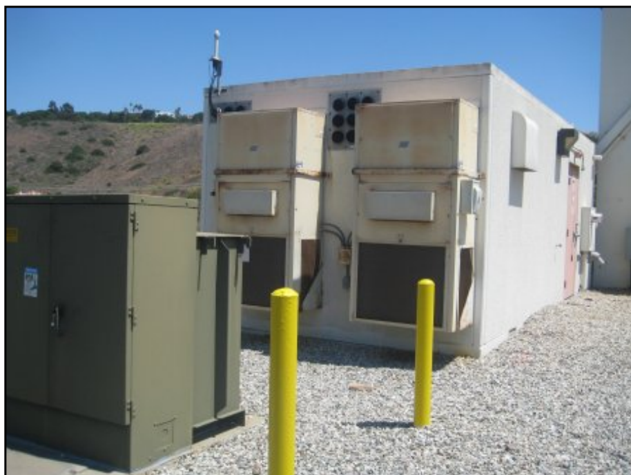
Former Emergency Generator Enclosure
