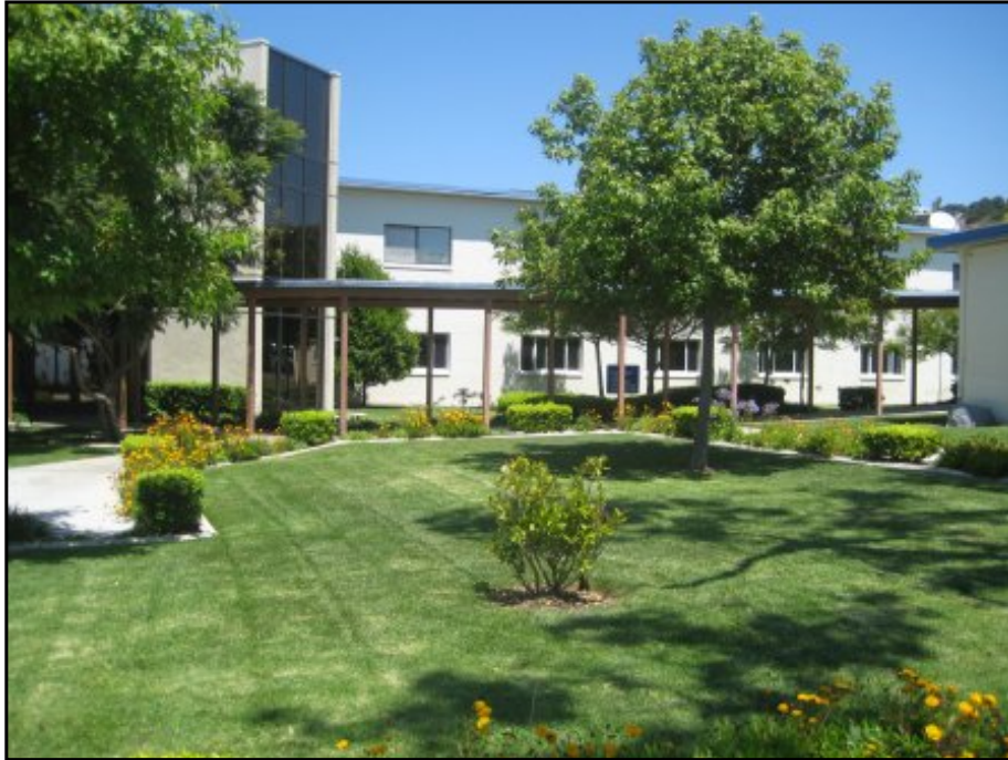
City Hall Entrance
