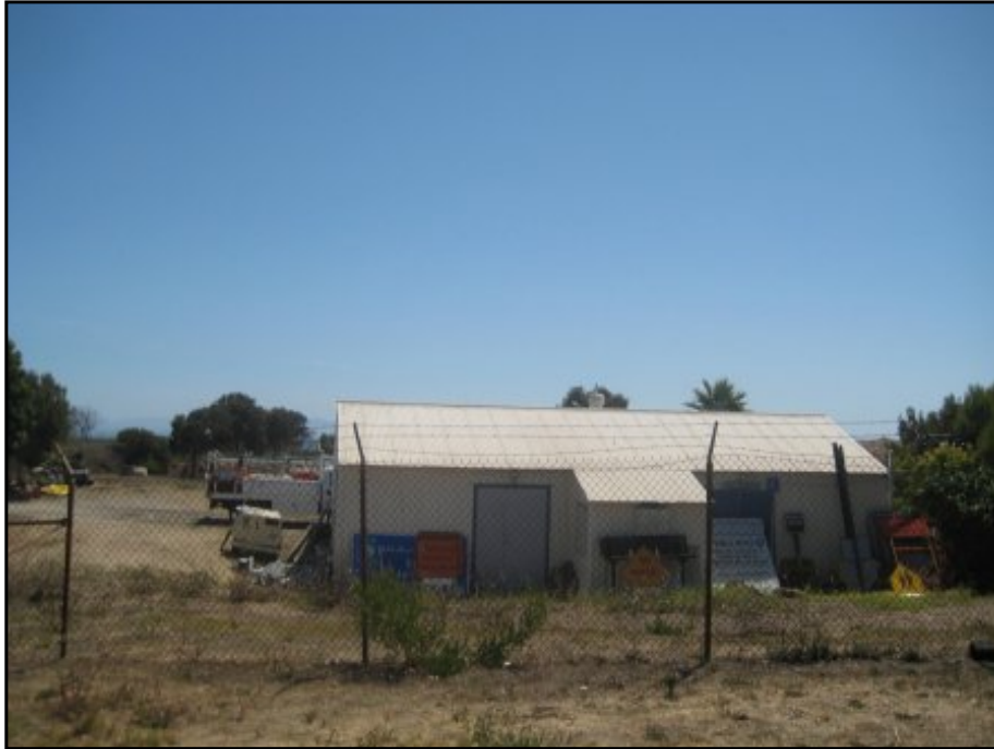
Generator Building (Traffic Control Equipment Storage) Building
