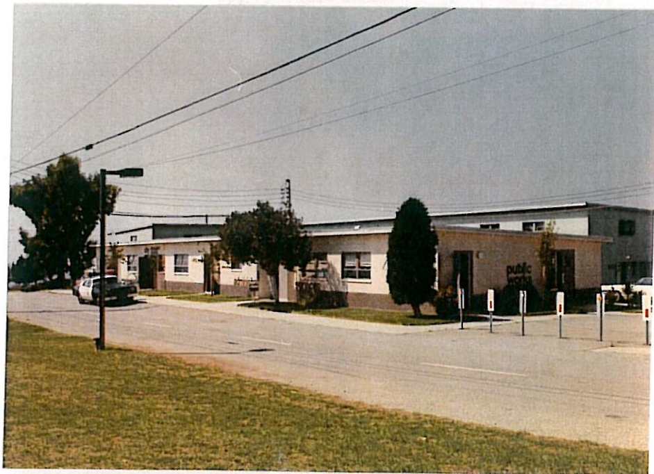
East and south sides of concrete block city office building on 4.6 acres
