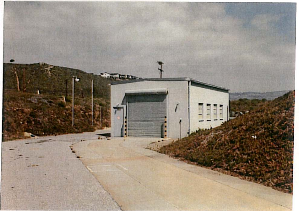
West end and south side of concrete block storage building near southeast corner of 4.6 acres
