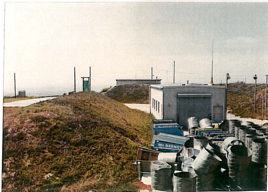
East end of concrete block storage building near southeast corner of 4.6 acres
