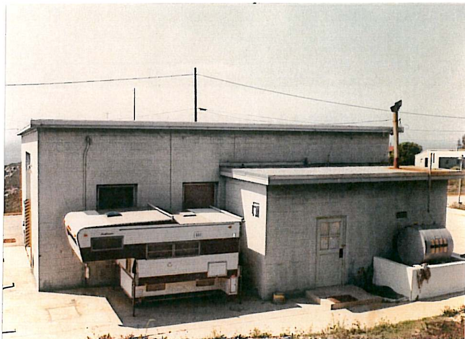
East side of former fire house
