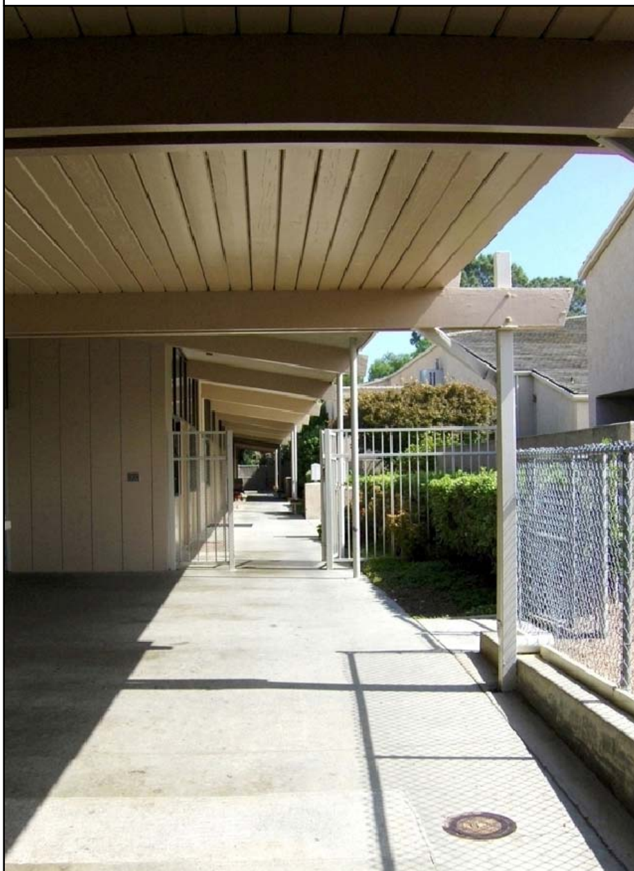
EXISTING SCHOOL WALKWAY
