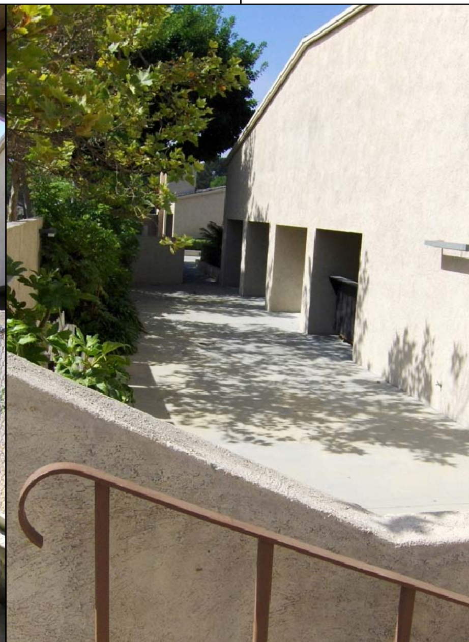
BARRETT HALL SERVICE STAIRS
