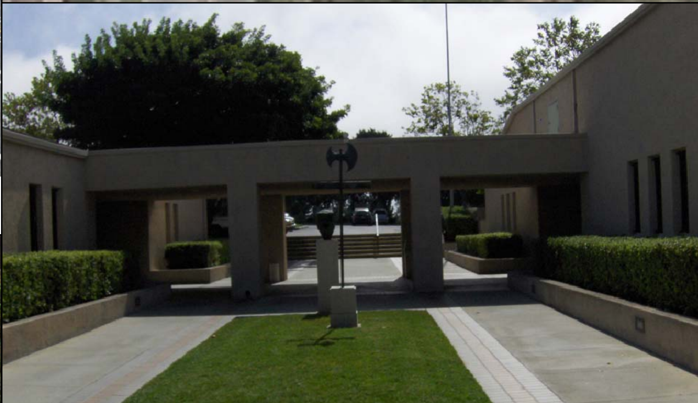
EXISTING CAMPUS ENTRY: INTERIOR VIEW
