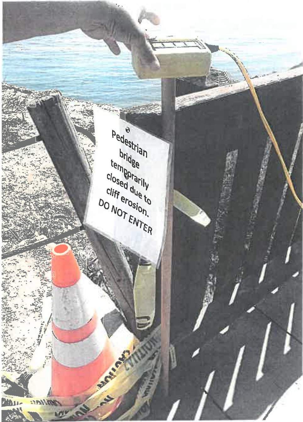
1 VIEW OF MANOMETER SURVEY TO VERIFY ELEVATION READINGS TAKEN FROM PRIOR SURVEY ON NOVEMBER 12, 2015
