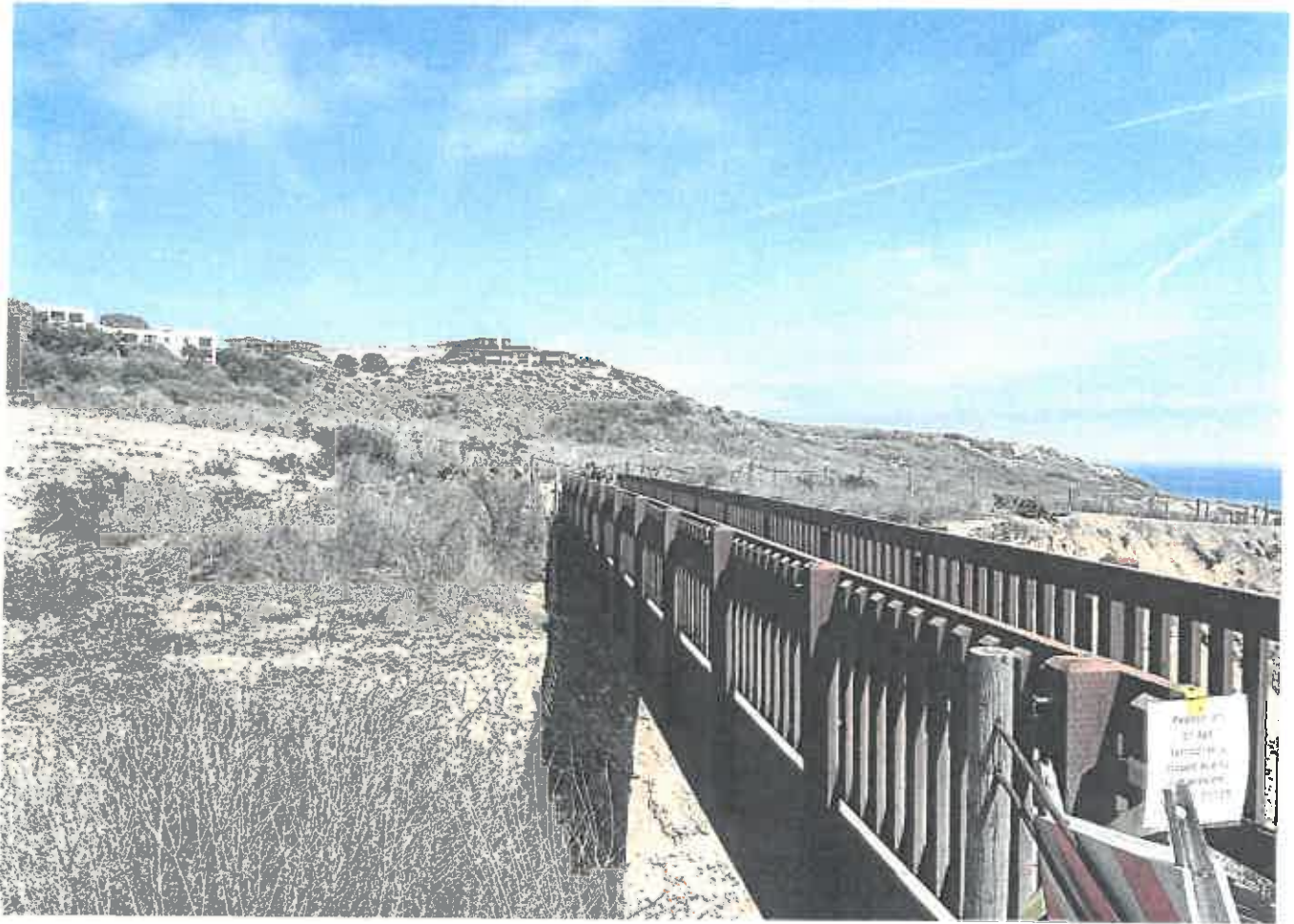
6 VIEW OF BRIDGE NO. 10 GIRDER TOWARD THE EAST ABUTMENT (NORTH)
