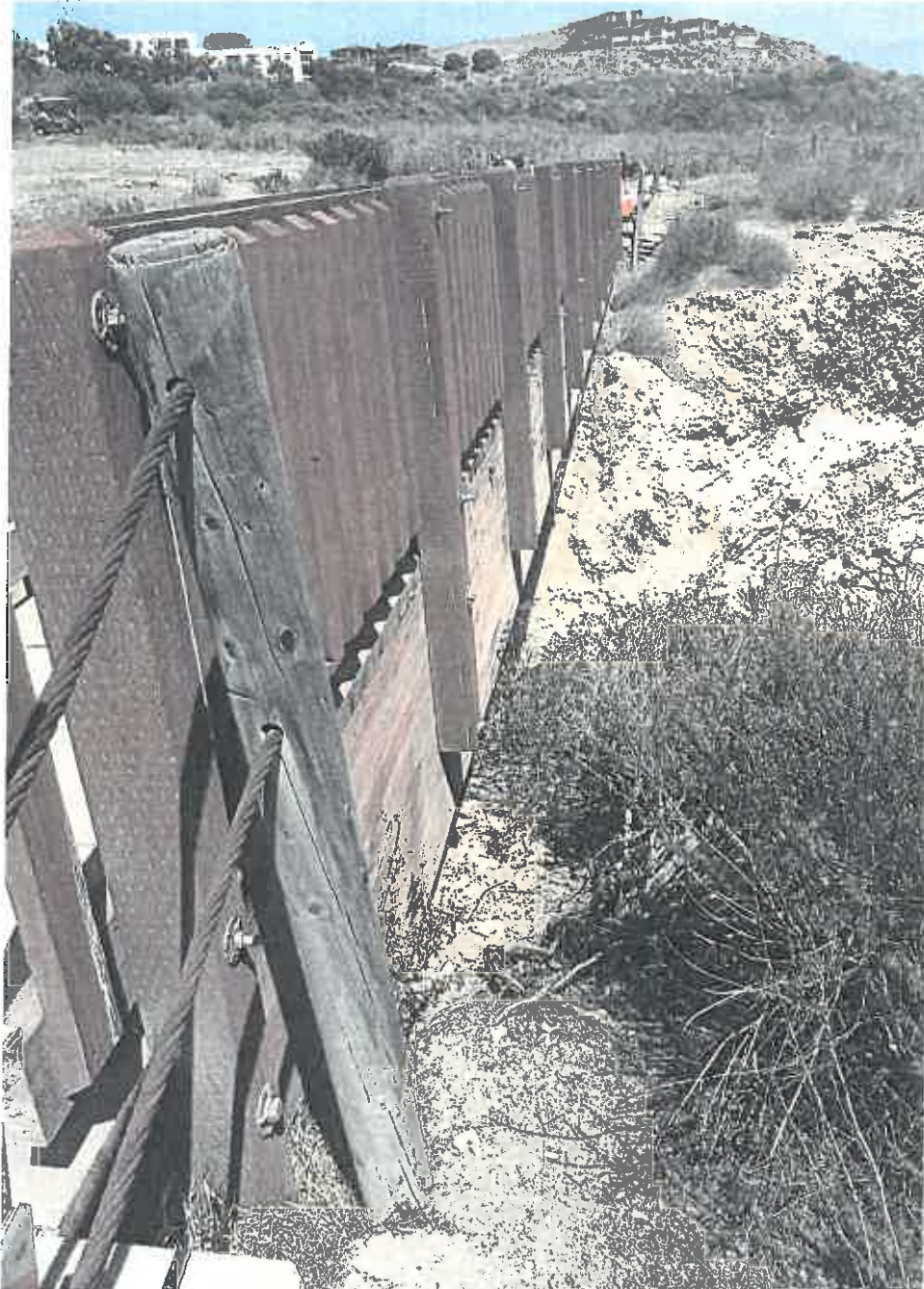
S VIEW OF BRIDGE NO. 10 GIRDER TOWARD THE EAST (SOUTH) ABUTMENT
