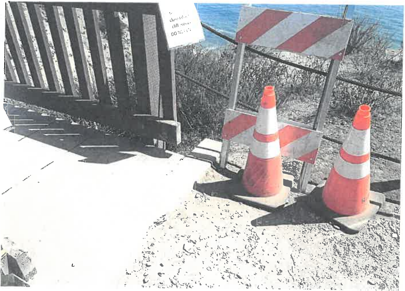
3 VIEW OF WEST ABUTMENT
