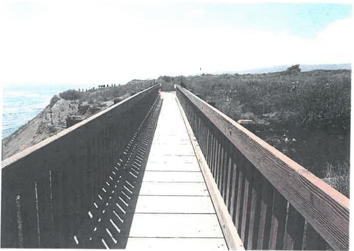
4 VIEW OF BRIDGE NO. 10 DECK SURFACE TOWARD THE WEST ABUTMENT
