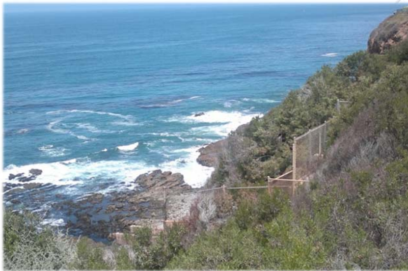
Figure 8.2: Outlet Structure to Ocean in Ocean West Drainage Area
