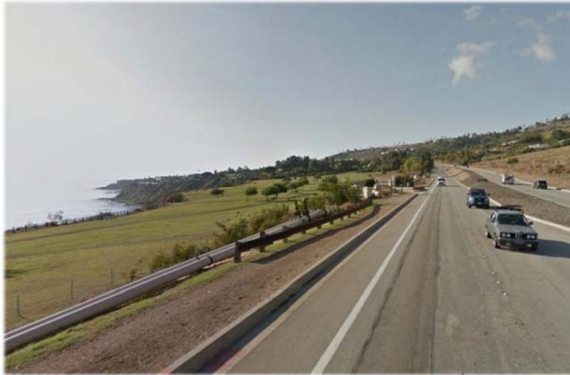
Figure 12.1: Palos Verdes Drive South along Landslide Area
